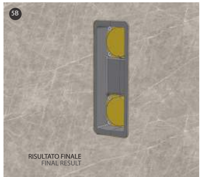
After removing the built-in box front cover, remove the cover exceeding the edge of the wall with a cutter.
